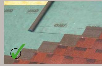
Tear off the old shingles and start building up with OSB, Underlayment and Cambridge Xtreme 9,5°.
