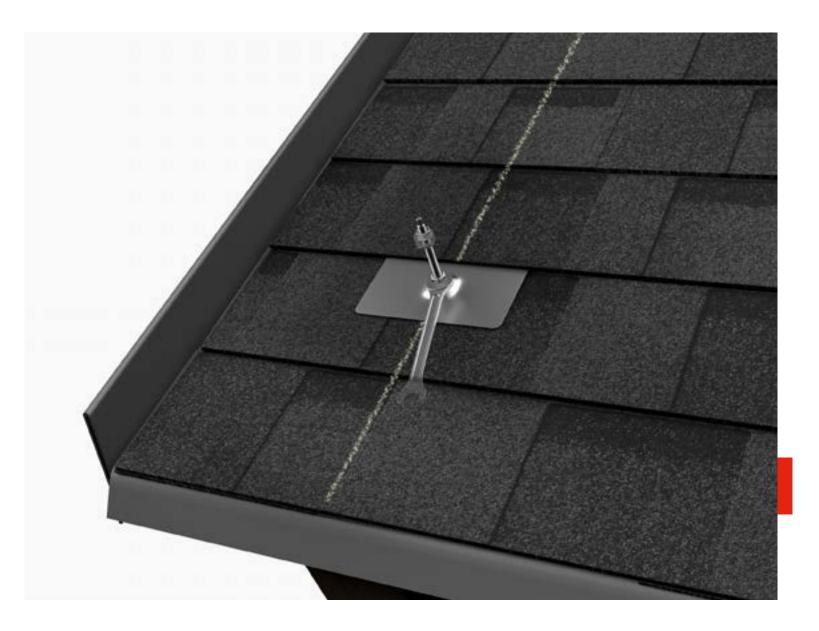
Install the mounting plate – adapter.
