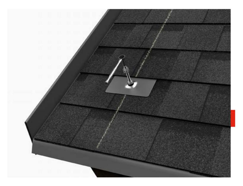
Seal and fasten lower serrated flange nut.
